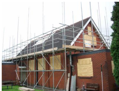
Tube and Coupler Scaffolds
