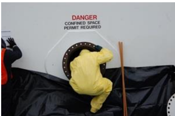
Figure 19 – Entering a Confined Space
