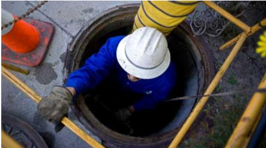
Figure 18 – Entering a Confined Space
