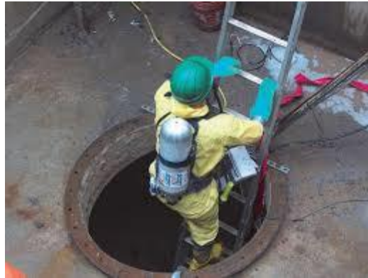
Figure 21 – Exiting from a Confined Space
