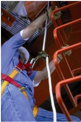
Figure 11 – Temporary rope line with rope grab
