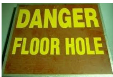
Figure 50 – Timber hole cover
