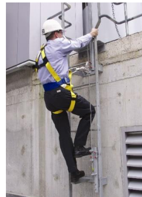
Figure 12 – Permanent wire line with wire grab
