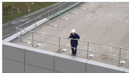
Figure 49 – Roof edge protection
