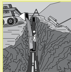
Figure 24: Example of an unguarded trench.
